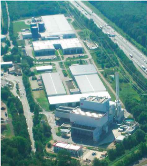
Figure 6. Hanover Waste Treatment Centre. MBT Plant (Background), Composting facility (Centre), Incineration Plant (Front)[9]
